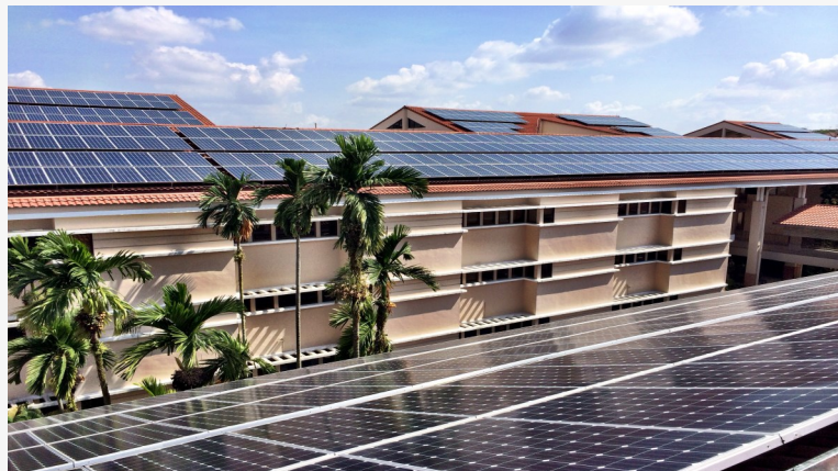
Solar installation on the Singapore American School. Photo: Sunseap Leasing
